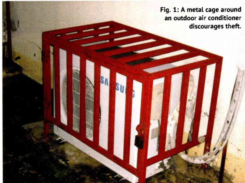
Fig. 1: A metal cage around an outdoor air conditioner discourages theft.
