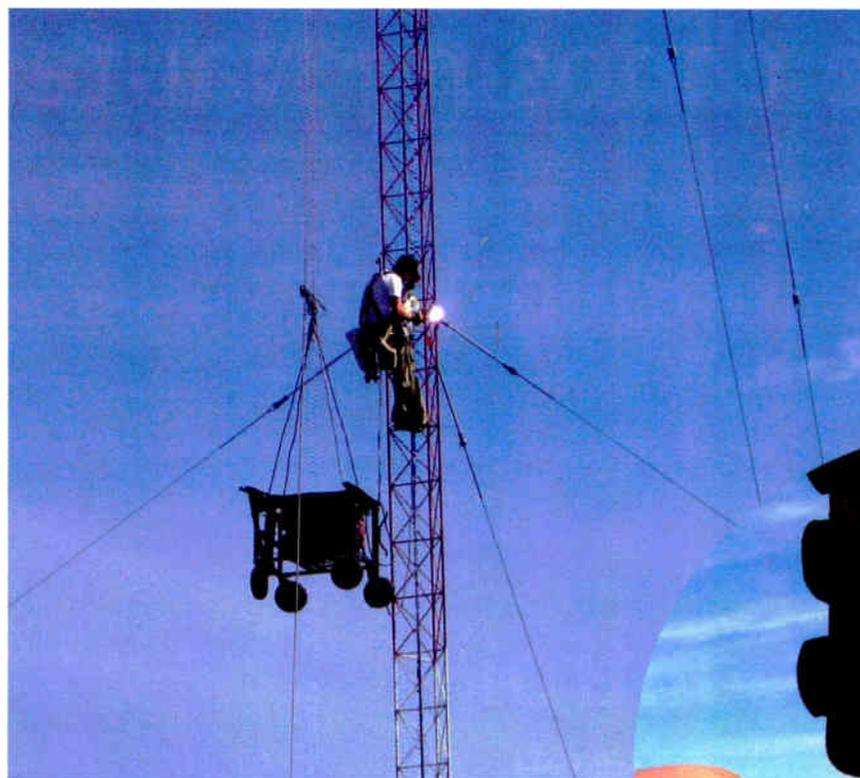
I have seen bonding straps that go around joints to remedy the problem. Others have run a heavy copper wire from the top to bottom of a tower. Those work, but a better approach is to weld the sections
