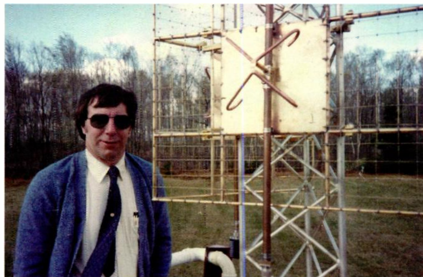
Below: Around 1976, Surette, under the tutelage of Ed Shively, designed this panel antenna, which was installed in North Bay, Ontario. At the time it was the most omnidirectional panel antenna on the market.
