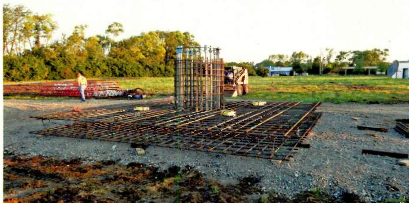
Rebar is put in for the new facilities.
