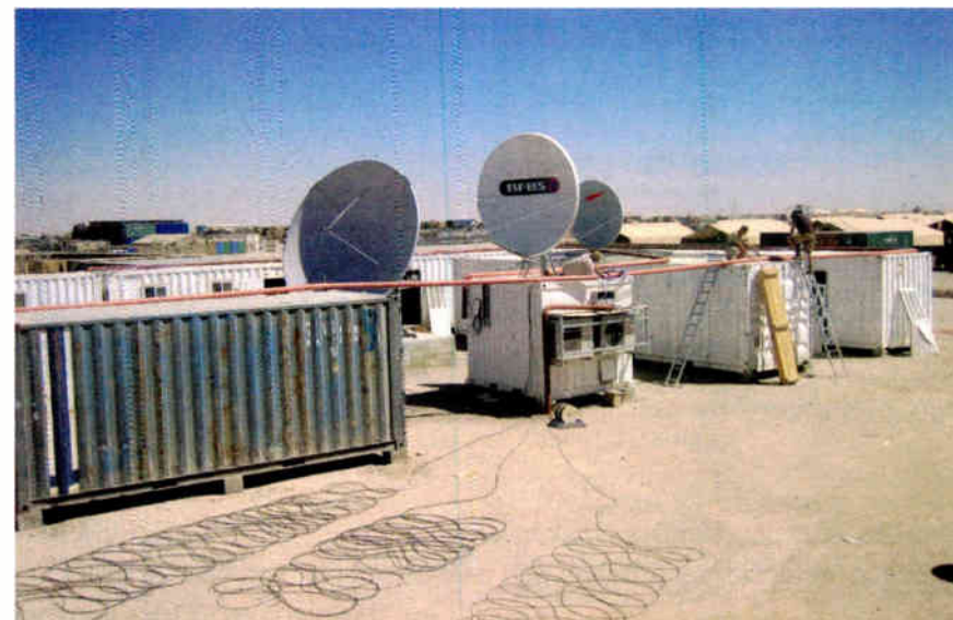
The studio complex under construction at Camp Bastion (known to American troops as Camp Leatherneck) in Helmand Province, Afghanistan. In the photo are the VSAT comms cabin and accommodation units. "There was over 10 kilometers of cable, audio, CAT-5, telephone, satellite, control laid around the site to two studios, two comms cabins, 14 accommodation units and a large office."
