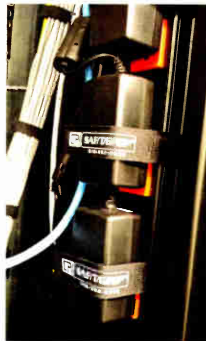
Fig. 3: Use this hook-and-loop strap to keep wallwart supplies in place.
