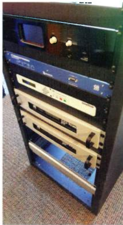
Fig. 1: Why not build that translator rack in your shop rather than on site?
