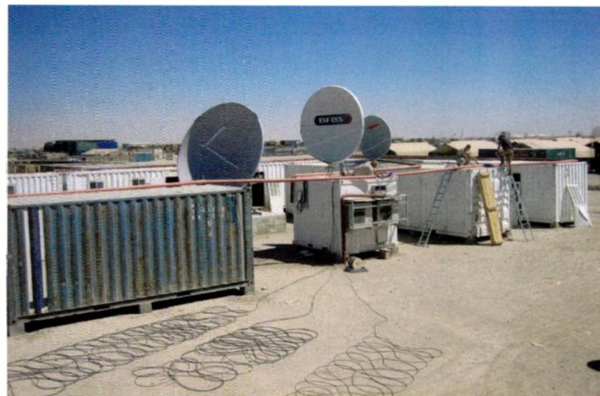
The studio complex under construction at Camp Bastion (known to American troops as Camp Leatherneck) in Helmand Province, Afghanistan. In the photo are the VSAT comms cabin and accommodation units. "There was over 10 kilometers of cable, audio, CAT-5, telephone, satellite, control laid around the site to two studios, two comms cabins, 14 accommodation units and a large office."
