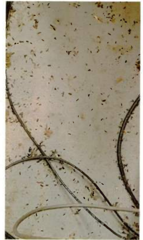
Fig. 4: Mouse droppings on the floor or the bottom of equipment racks are a dead giveaway your site has rodents.
