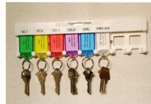
Fig. 5: An inexpensive, wall-mounted transmitter site key holder. Each key is identified not only by station but also with the address.
