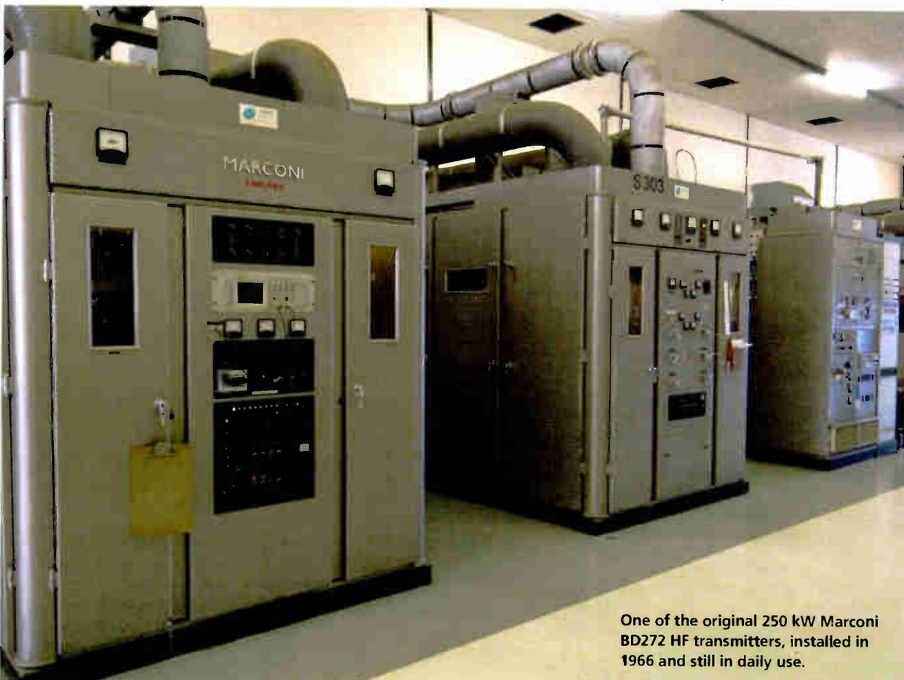
One of the original 250 kW Marconi BD272 HF transmitters, installed in 1966 and still in daily use.
