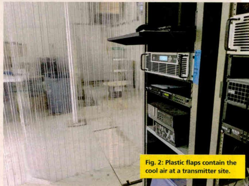
Fig. 2: Plastic flaps contain the cool air at a transmitter site.
