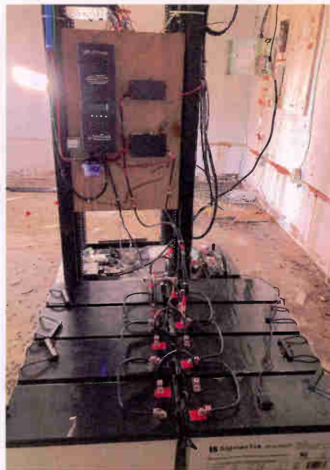
Above: Bird's-eye view of the solar panels atop the KUHS transmitter building. Right: A bank of eight Sigmas Tek 200 Ah sealed lead acid batteries provide enough reserve power to run the transmitter site for about a week.
