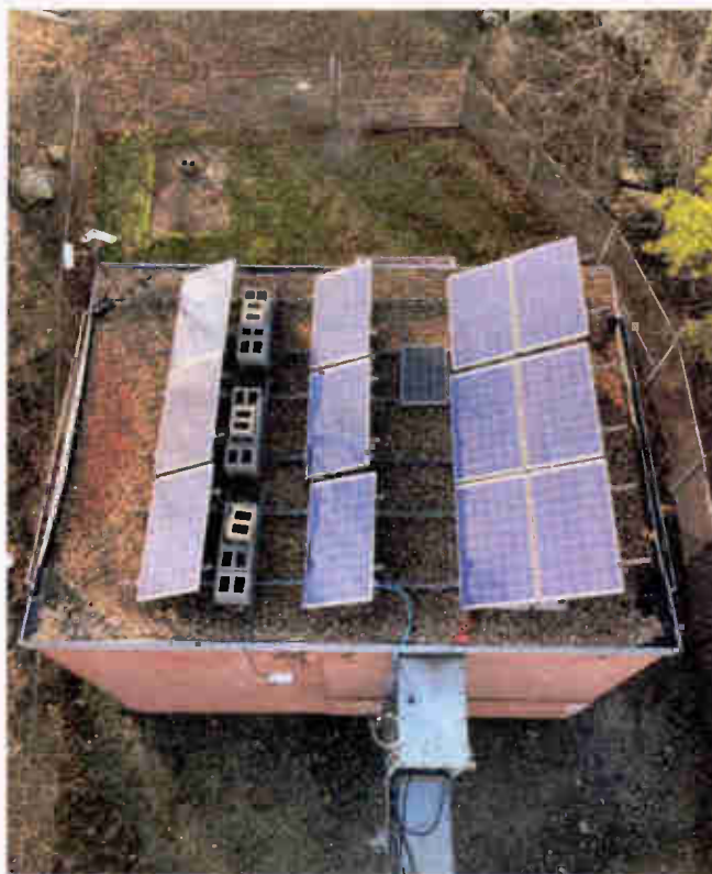
Above: Bird's-eye view of the solar panels atop the KUHS transmitter building. Right: A bank of eight Sigmas Tek 200 Ah sealed lead acid batteries provide enough reserve power to run the transmitter site for about a week.
