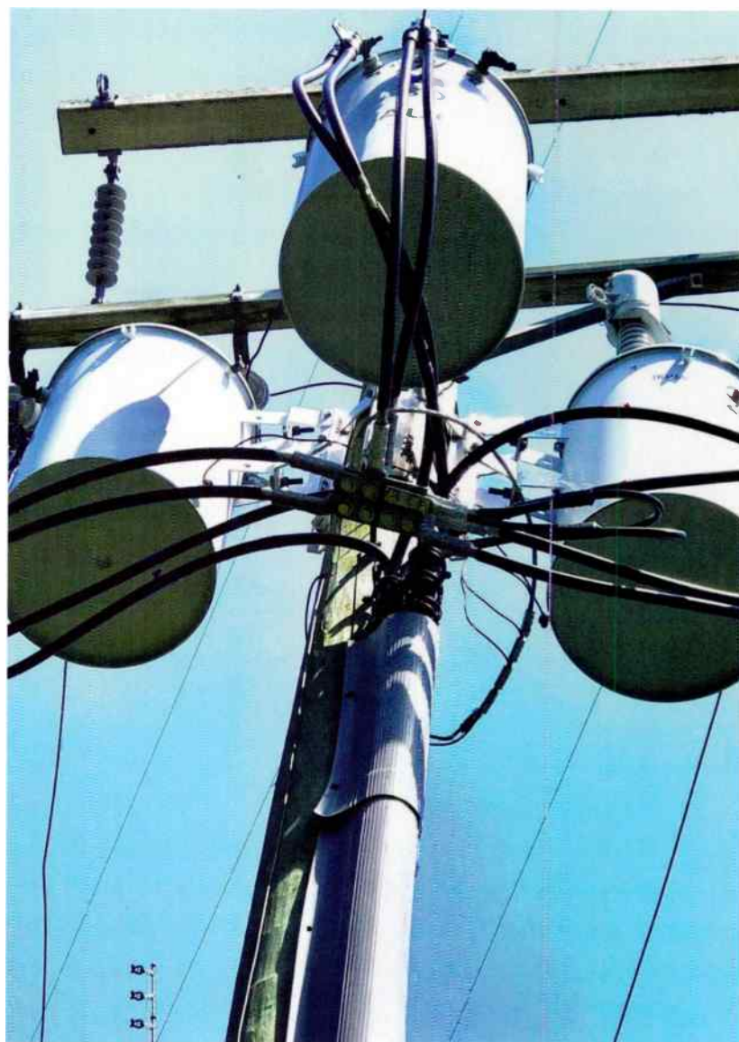
Above Left Fig. 2: Closed delta secondary feed
