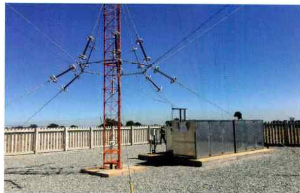
Below Fig. 12: Base region geometry of a six-wire flared skirt, upper image, and a flared skirt replacing conventional skirt due to instability in icing conditions, bottom image.
