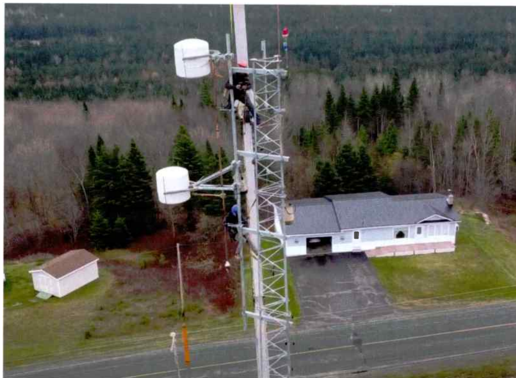
Above Installation work in progress.
