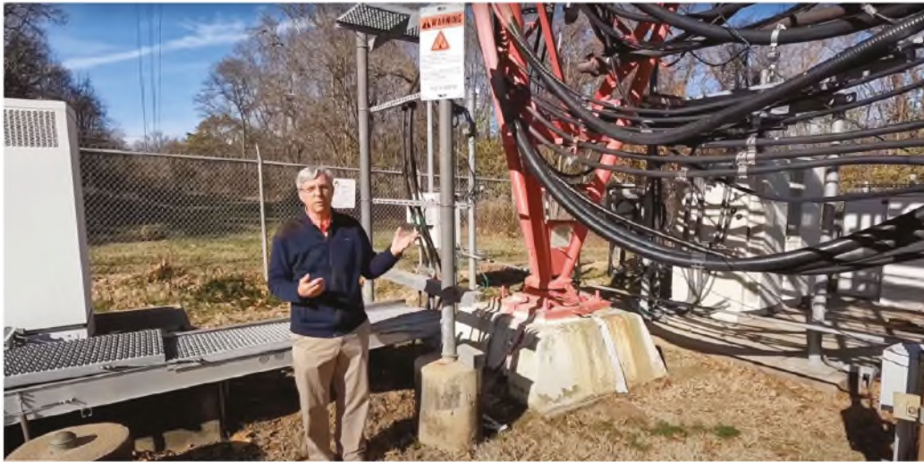
Above Joe standing at the tower base.
