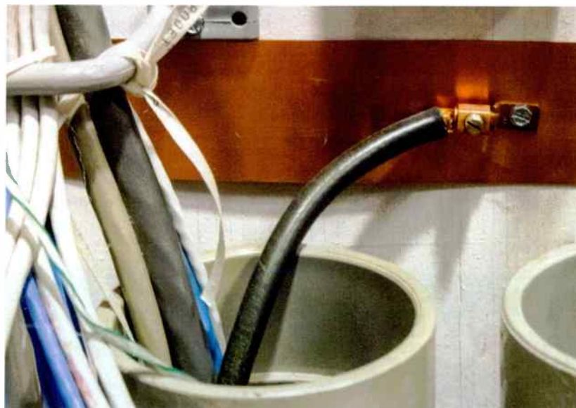
Above Fig. 6: Don't use a ground cheater.
