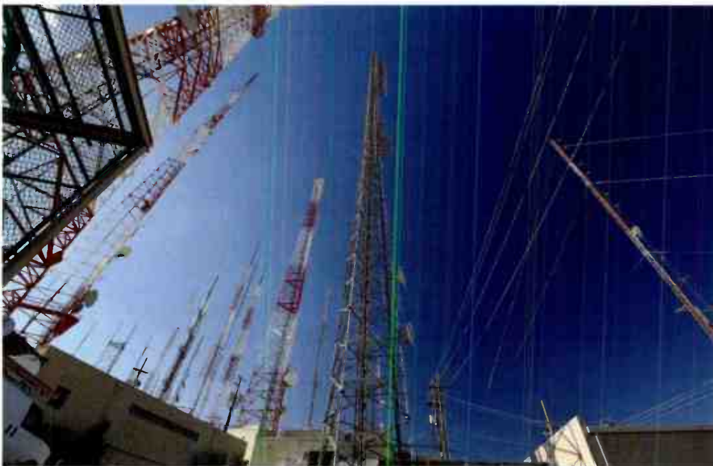
Below The new tower is at center; its crowded RF environment is evident in this photo.
