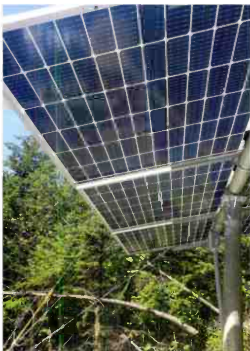
Left The underside of the panels can receive energy from reflected light.
