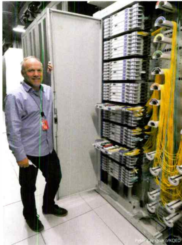
Left Dave Hansen with cabling.
