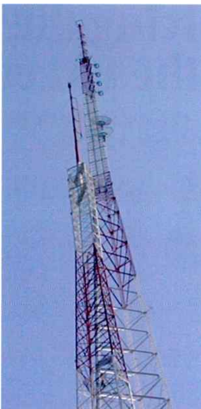
Above The "new" 500-foot tower is shown next to the older 360-foot structure. Note the identical four-bay main and aux antennas.
