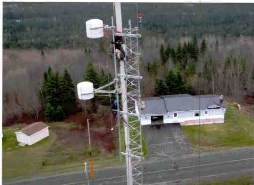
Above Installation work in progress.
