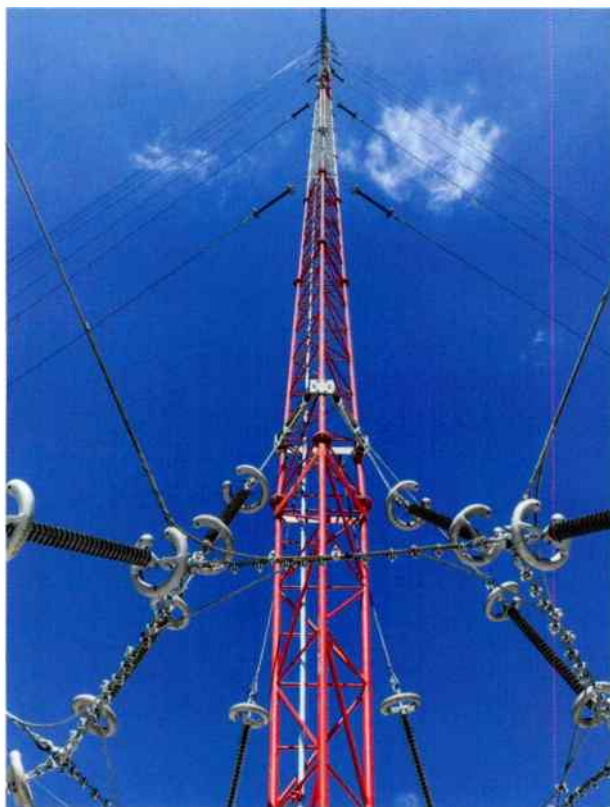
Left Fig. 2: A photo of the 140m grounded, flared skirt-fed Dak Lak tower designed for 2 x 200 kW diplexed operation.
