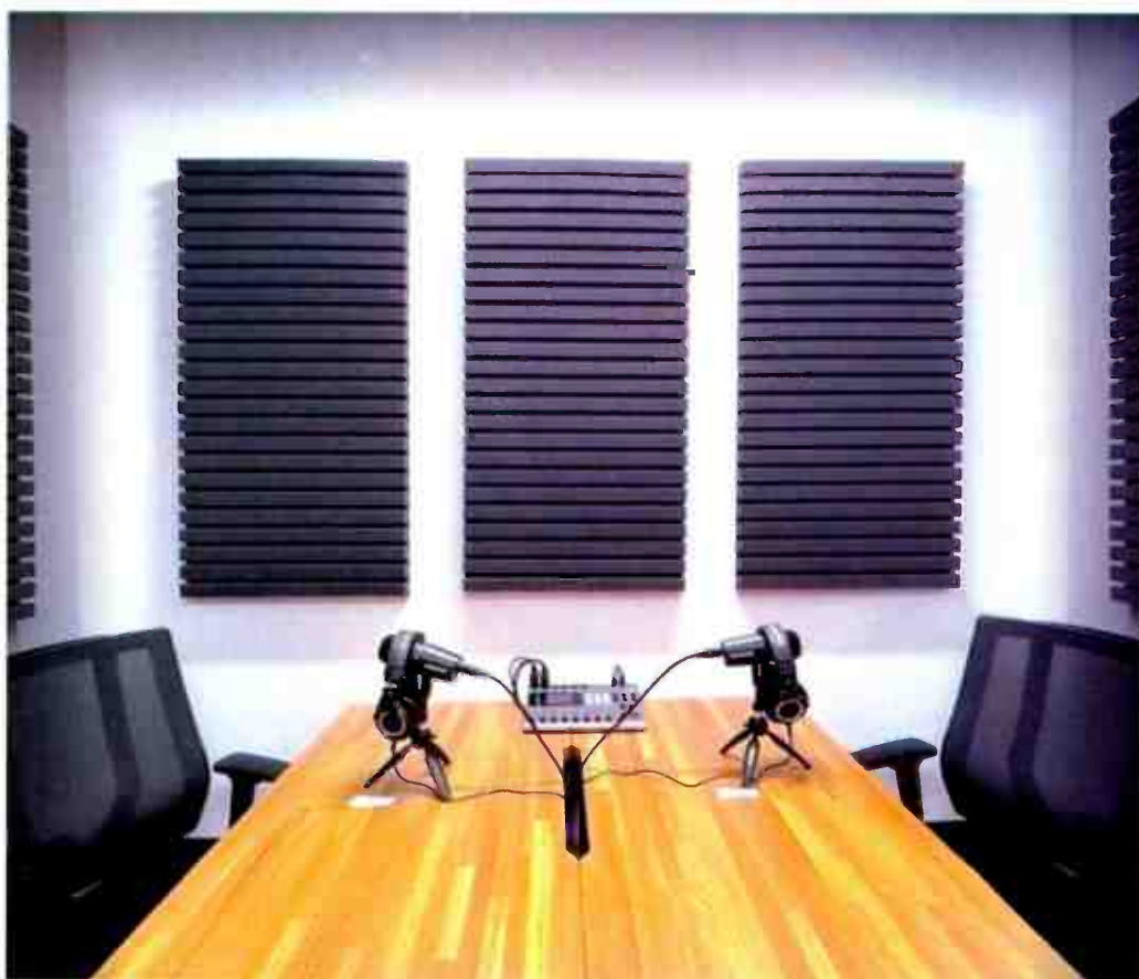
Above Auralex Studiofoam T absorption panels installed in podcast studio.
