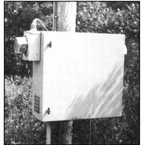
A typical equipment cabinet for a buried cable system along a road.
