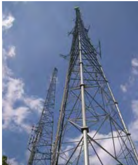
Figure 1. Two towers are located at KPTM's downtown Omaha studios. A lightning strike to one of these towers followed waveguides directly into the adjacent studio building.
