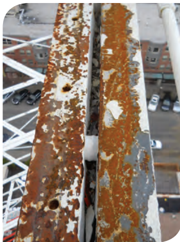
If your tower has LBP, develop a Lead Control Plan to address the situation before it becomes a problem.
