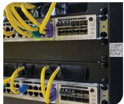
Fig. 5. QR codes on the rack frame link to a system diagram.
