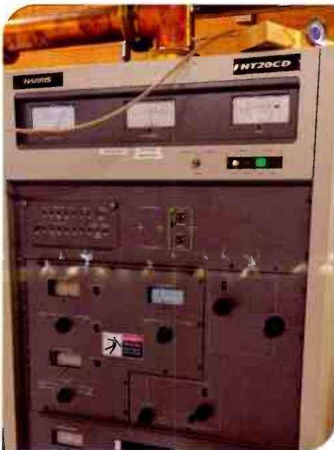
The Harris HT series is a common tetrode-based transmitter.
