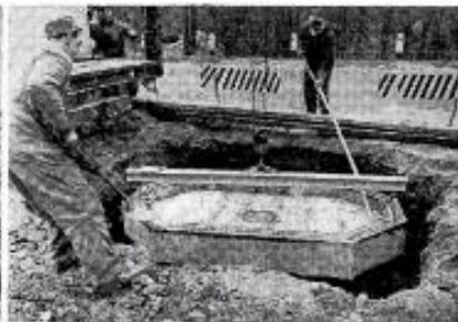
Lower manhole vault ...
