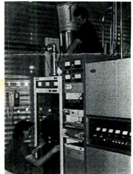
Installing the new transmitter at Z99
