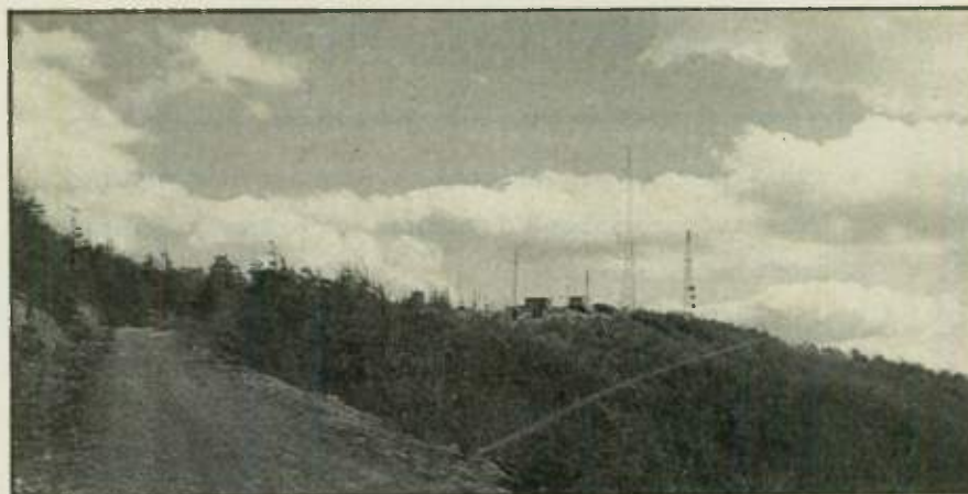
WMIT approach and towers
