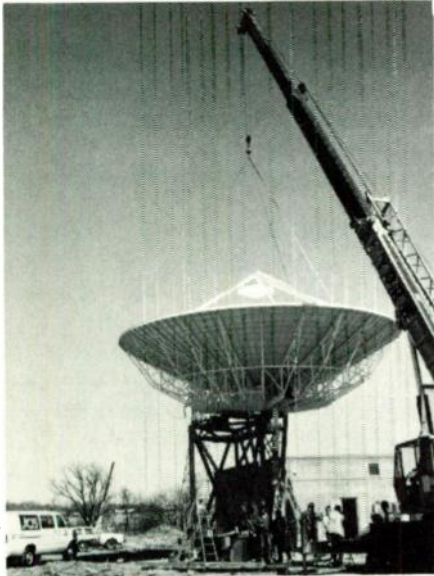
Two-ton, 36-foot satellite dish is lowered in to place on the site of the ACTS station
