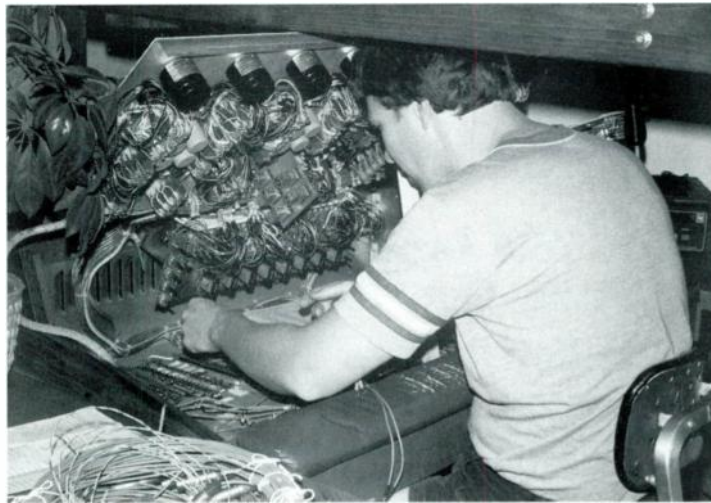
Ken Boone wires the "We Kids" under-the-bed studio.
