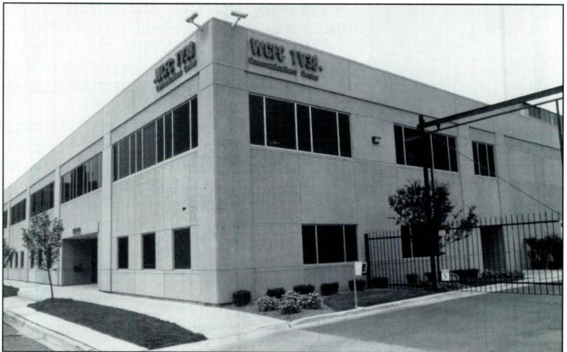
TV38's Communications Center is a 42,000 square-foot facility located in a growing area of downtown Chicago.
