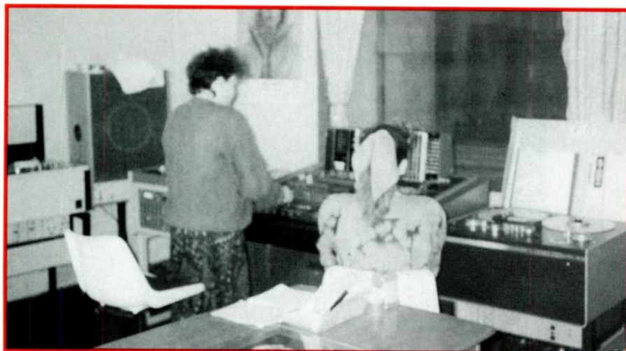
Most of the control room operators in the Commonwealth of Independent States are women.
