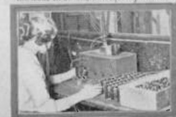
Above shows Miss Gay Garrity soldering the leads of an audio frequency transformer.
