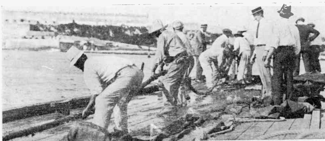
Running the barge under the cable by man-power
