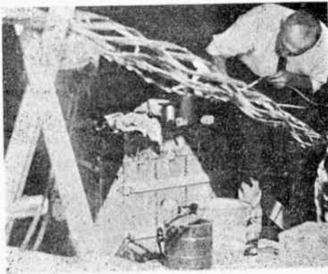
Bruno Trehes splicing a good piece into the mashed cable
