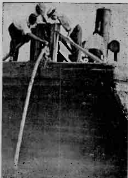
Running the cable through the pulley on board the barge
