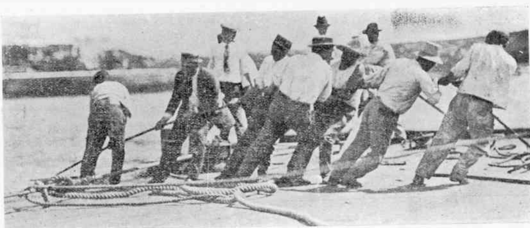
Dragging the cable on board the barge
