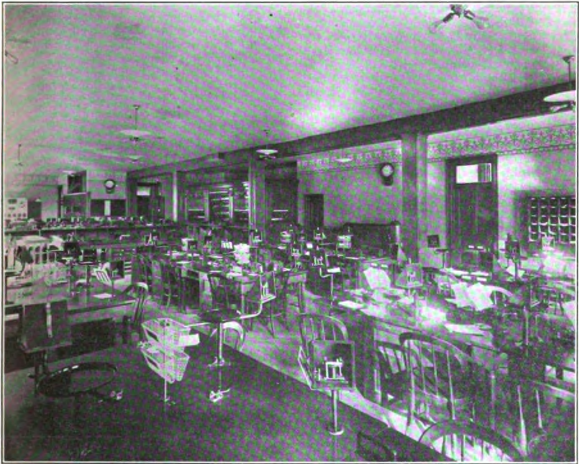
GENERAL VIEW OF THE OPERATING ROOM, POSTAL TELEGRAPH CABLE COMPANY, BUFFALO, NEW YORK.
