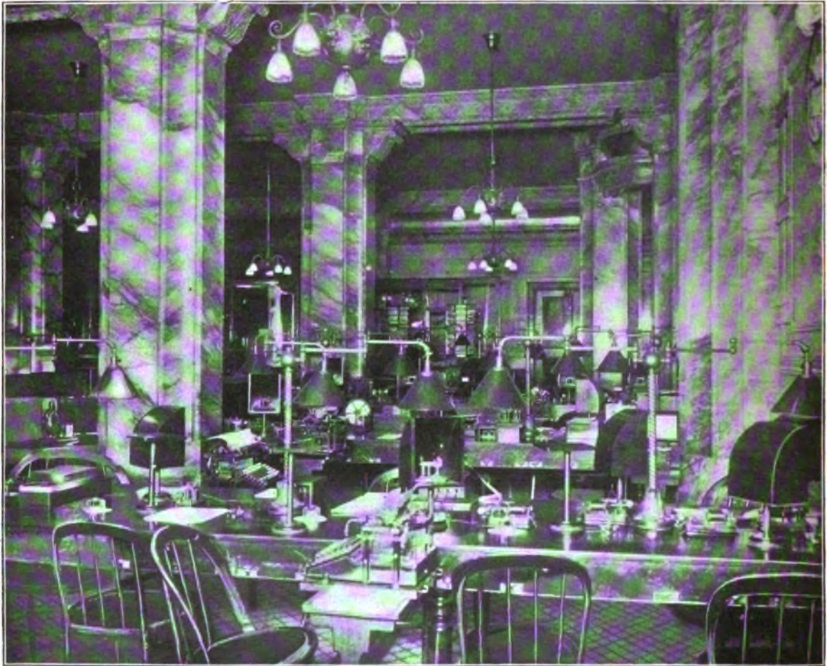
GENERAL VIEW OF THE OPERATING ROOM IN THE NEW OFFICE OF THE POSTAL TELEGRAPH-CABLE COMPANY, BUFFALO, N. Y.
