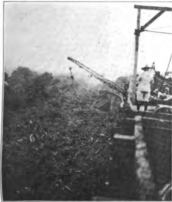
LAYING THE CABLE ALONG THE PANAMA RAILROAD WITH A DERRICK CRANE.
