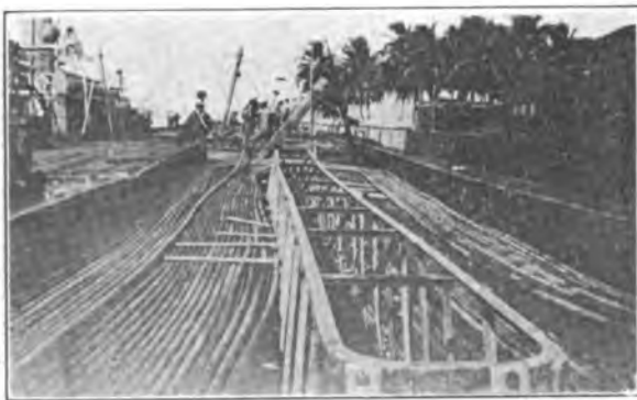
VIEW SHOWING CABLE COILED ON CARS.
