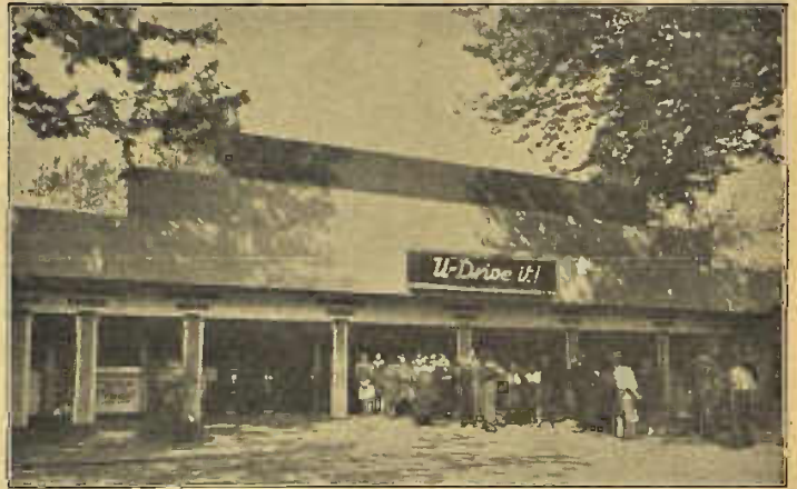
ONE OF THE NEW FEATURES in Belmont Park, Montreal, is the new 20-streamlined-car Skooter housed in a new building 60 by 80 feet, constructed by the Belmont Park Company. Modernized front was designed by General Manager Rez D. Billings.
