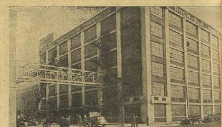
DERRICK AND STEEL are symbols of progress. Above is a scene taken at the Rock-Ola factory, Chicago. Workmen are constructing an aerialway to link the main building to an auxiliary building across the street.
