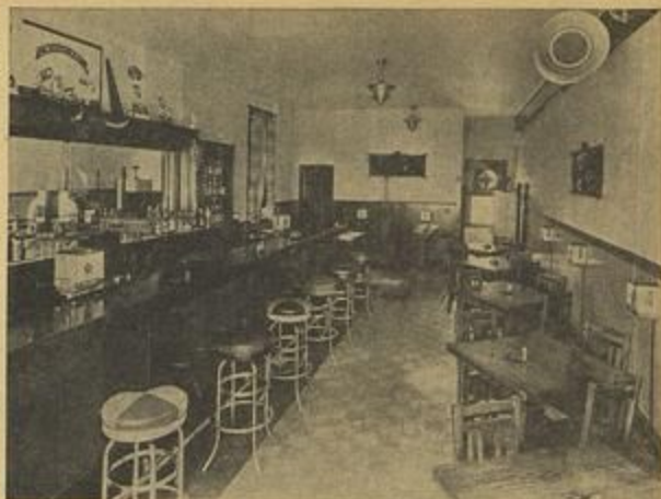
THERE'S ALWAYS MUSIC WITHIN reaching distance in the Bonfanti Buffet, St. Louis. Public Sound Systems has installed Keeney wall boxes at frequent intervals on the walls and bar.
