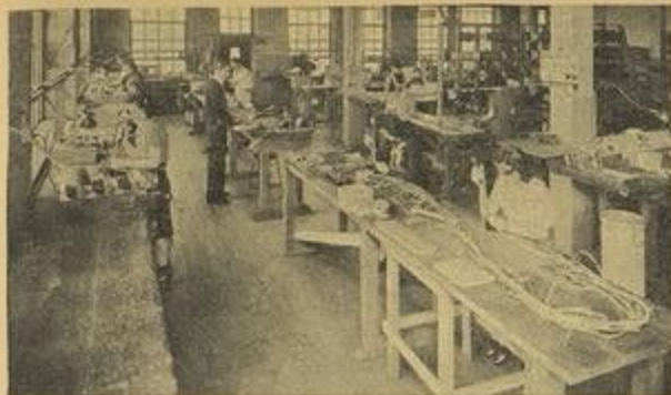
LARGE WIRING DEPARTMENT of O. D. Jennings & Company, where skilled employees are busy with the wiring of the Jennings telephone music systems.
