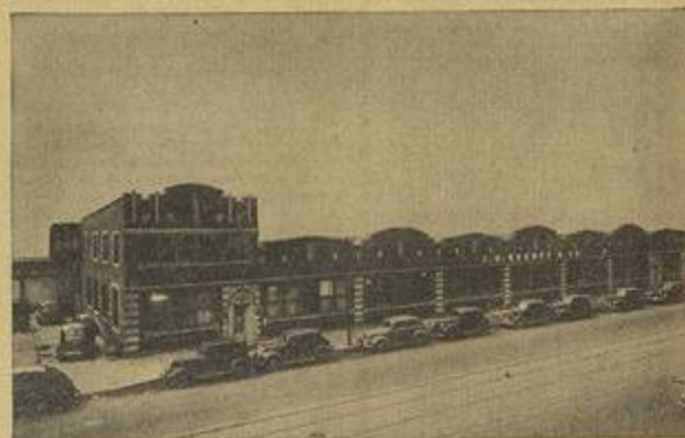
NEW J. H. KEENEY & COMPANY FACTORY in Chicago. "It is one of the most modern coin machine plants in the industry," declares William Ryan, Keeney sales manager. Full production on current Keeney machines has already begun in the new location.
