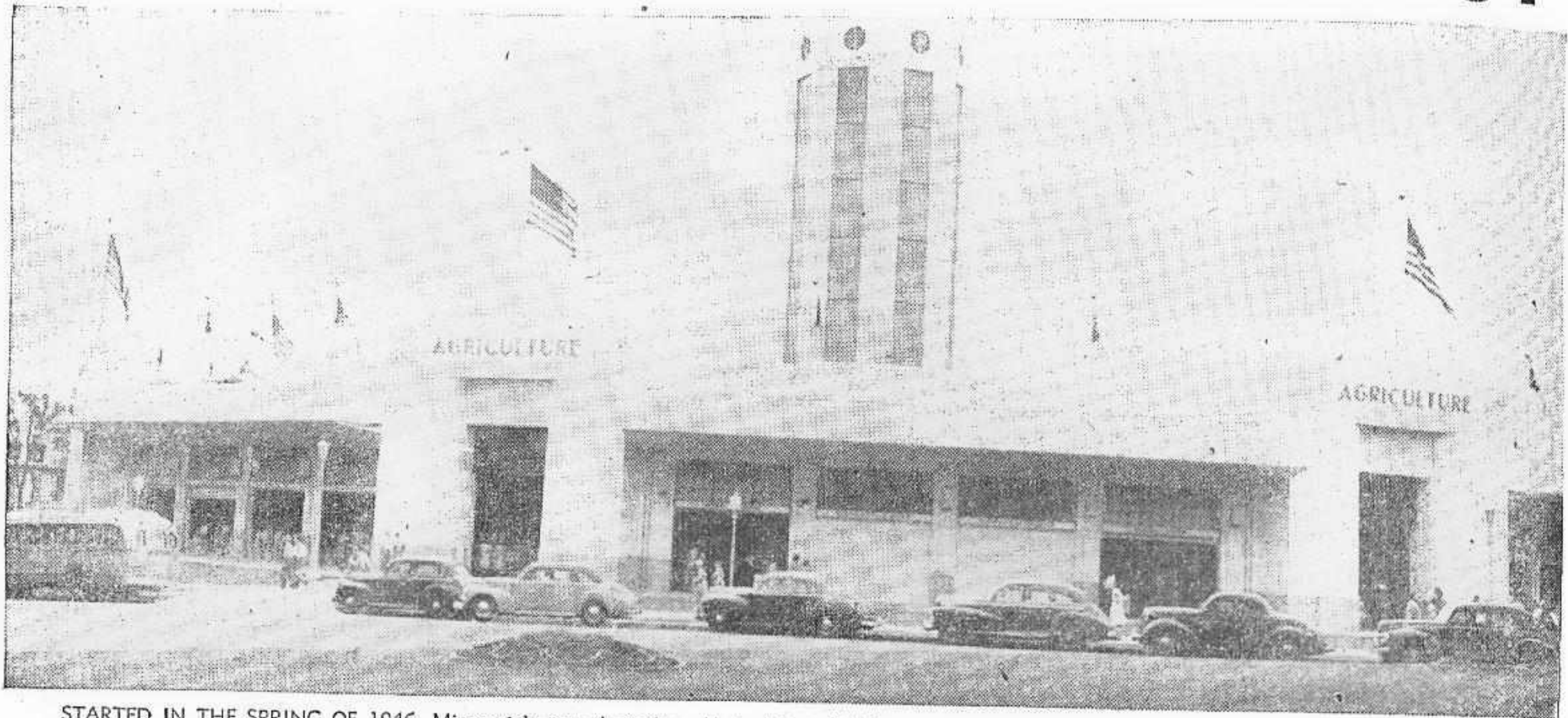
STARTED IN THE SPRING OF 1946, Minnesota's new Agriculture-Horticulture Building was completed in time for the 1947 fair. The design, utility and appearance of the structure has drawn much praise from fair executives.
