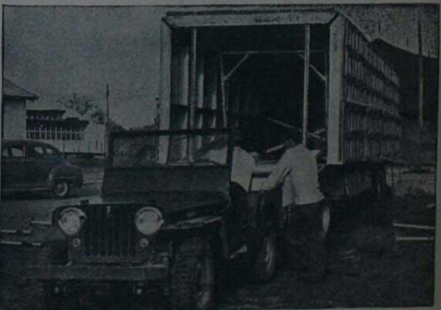
ONE OF THE GREATEST FEATURES of the trucks are their mobility. Easily moved into position by jeep and wheeled out of position with equal smoothness, the problem of throwing up the tent is reduced. Interior of the trucks will be utilized for storage of equipment.
