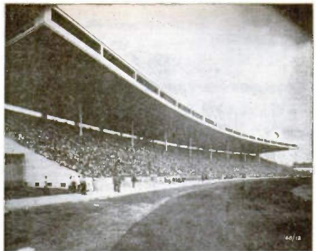
Sweeping view shows how stand's design and construction enables perfect vision from almost every point. Huge battery of lights may be noted at the edge of the roof's center.
