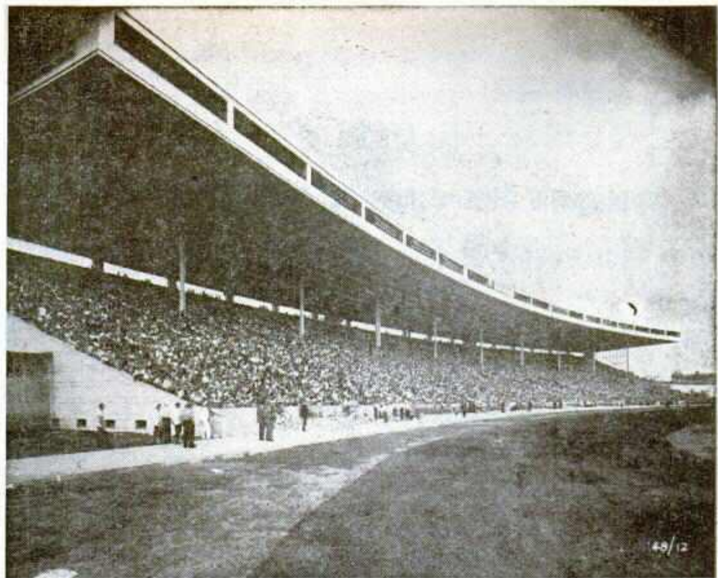
Sweeping view shows how stand's design and construction enables perfect vision from almost every point. Huge battery of lights may be noted at the edge of the roof's center.
