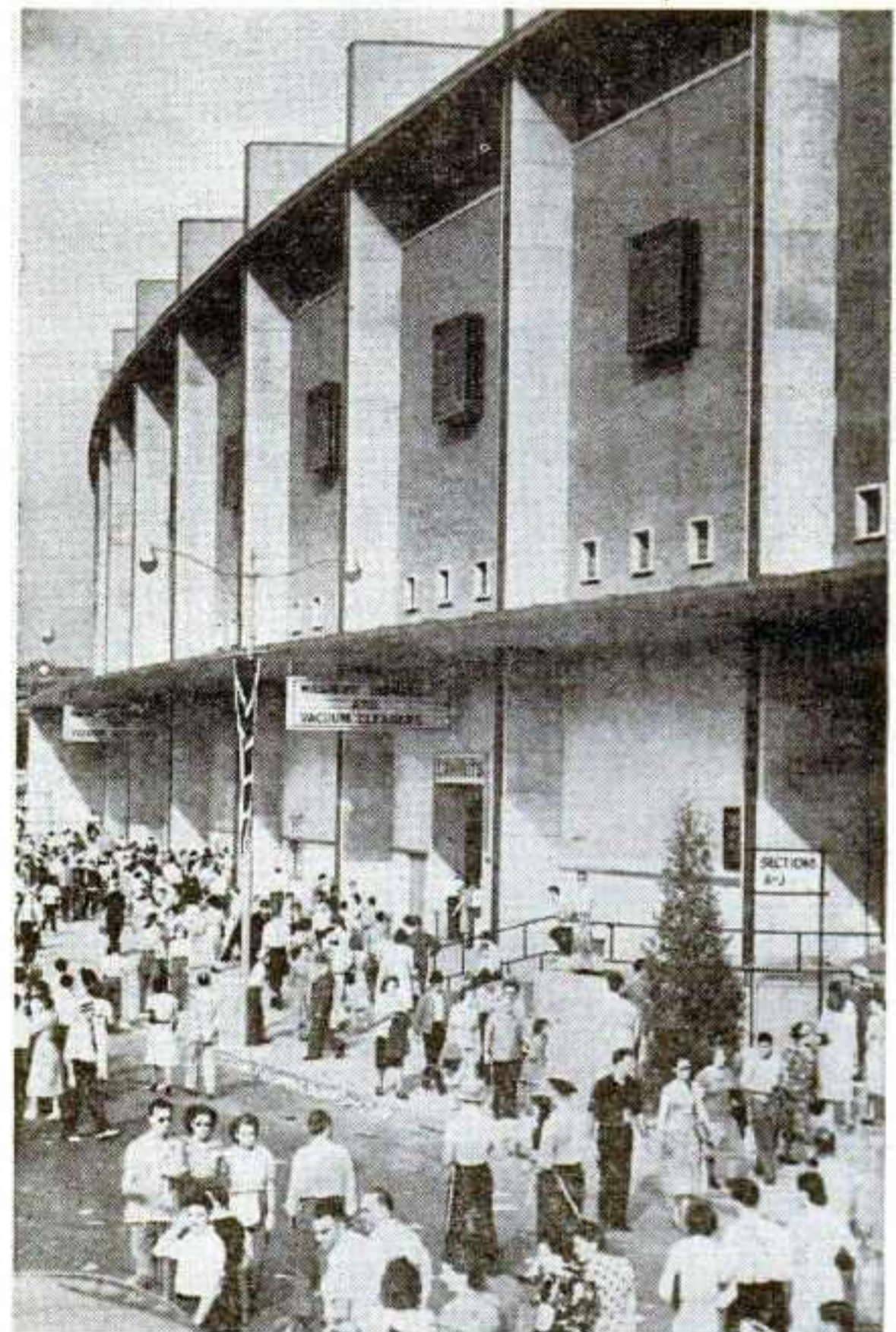
Commodious eateries, large exhibit area, storage space, and rest and dressing rooms are provided underneath the rising tier of seats. Portion of stand's front pictured shows an entrance to exhibit hall.
