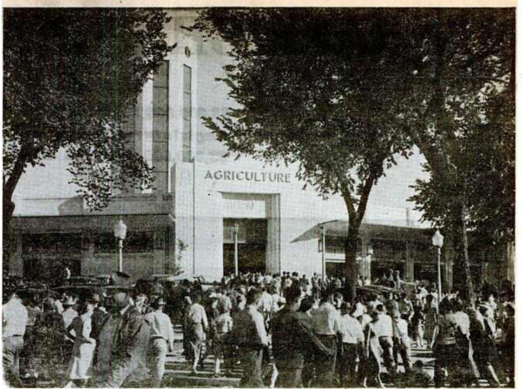
Minnesota State Fair this year drew an all-time high attendance of 905,563 persons. Picture shows a typical section of a 1950 fair crowd near the Agricultural Building.
