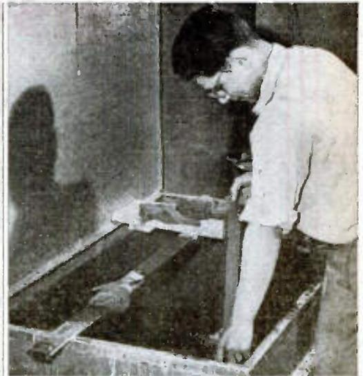
ANOTHER ASPECT of preventive maintenance is cleanliness. Using a cleansing solution and a good-size tank or tub as a degreaser such as is used in industrial plants, the operator can dunk both small and large juke parts equally well. An easy brush-off after removal from the solution usually serves to whisk away undesired accumulations of dirt and grease. Here a Seeburg record assembly is being cleansed of foreign matter which could affect disk delivery.
