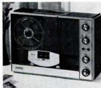
Model 2075 identifies the new Ampex tape recorder/player billed as "a unique combination of living-room furniture styling and portability." The unit is cabineted in oiled walnut, has built-in amplifier and speakers and features automatic threading and reversing, permitting play of both sides of a stereo tape without reversing or handling. List price is \$529.
