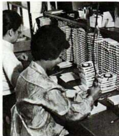
SPLICING CONTINUOUS LOOP tape and sealing the cartridges and cassettes is handled by a separate staff.
