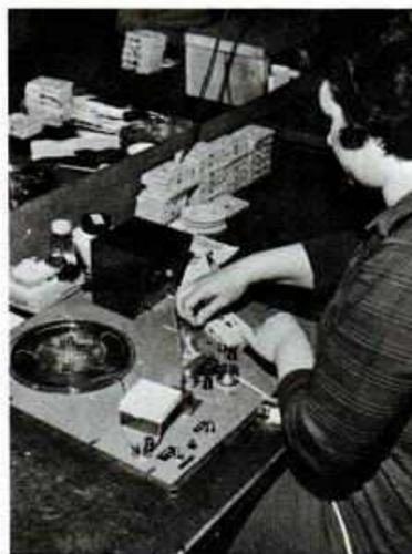
CLOSE-UP of the winding procedure done on A&B's automatic unit, which cuts the tape at the end of each complete cartridge. Pancake generally contains 10 cartridges.
