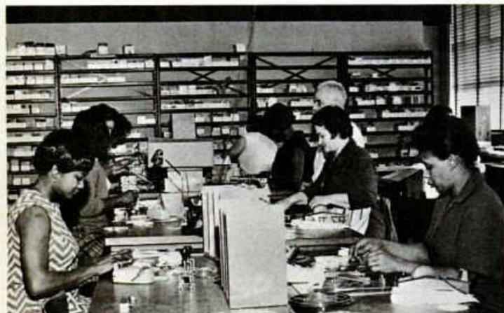
WINDING TAPE INTO CARTRIDGES from the pancake reels duplicated on the slaves is the next phase of A&B's operation. The Bell Sound division employs some 60 workers, although that number occasionally rises to 90.
