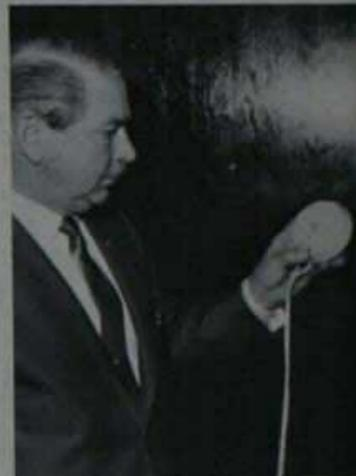
JOHN PENTECOST, Rowe engineer, examines the transducer, a device that mounts in walls, ceilings and even table tops, and acts as a transmitter of sound. Rowe is introducing the device with its new Music Master jukebox.
