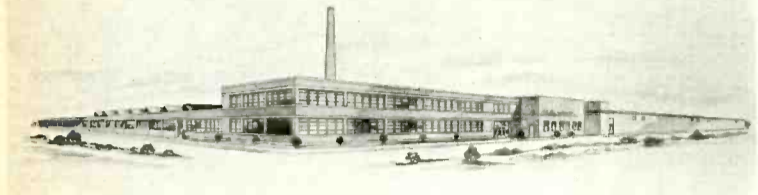
BALLY Manufacturing Corp.'s main plant, as shown in this artist's rendering, now extends for a full block along Belmont Avenue in Chicago. A new addition on the east side furnishes 50,000 additional square feet of manufacturing space. The firm also occupies two buildings across the street from the main plant.
